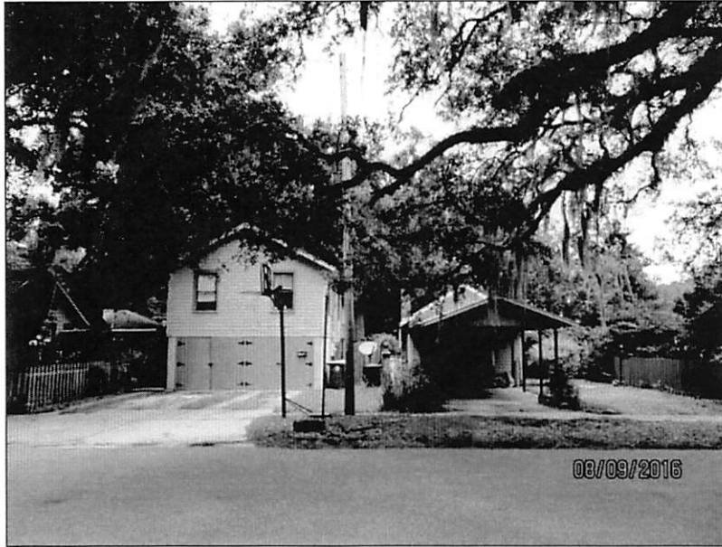
Rear yard accessory structures north along Glendale Street.
